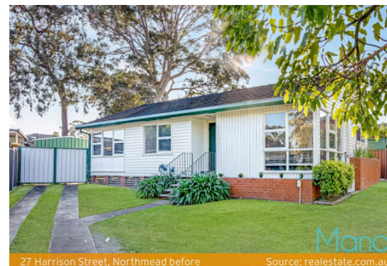
27 Harrison Street, Northmead before
