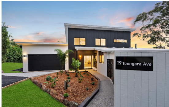
19 Toongara Avenue, Bateau Bay after Source: CoreLogic
