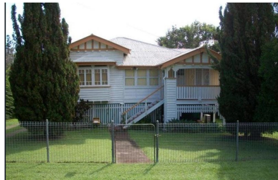
Talford Street on The Range before Source: CoreLogic
