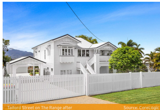
Talford Street on The Range after Source: CoreLogic
